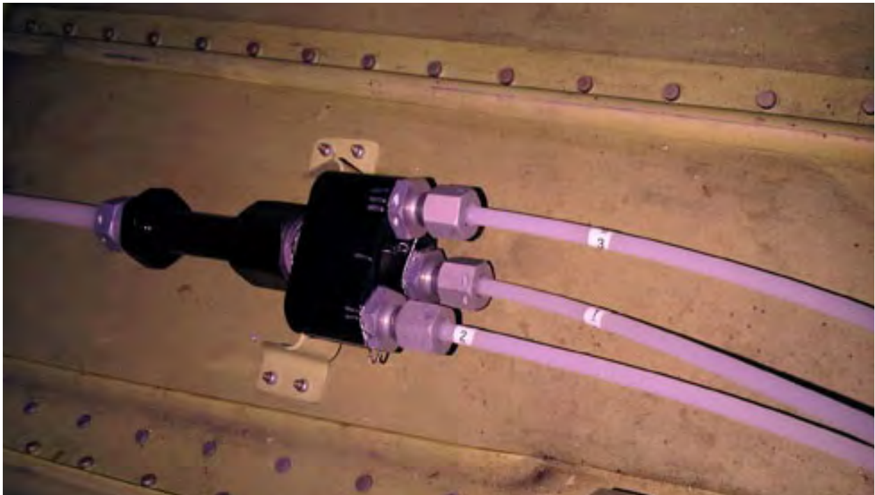
The tail proportioning unit is installed.
