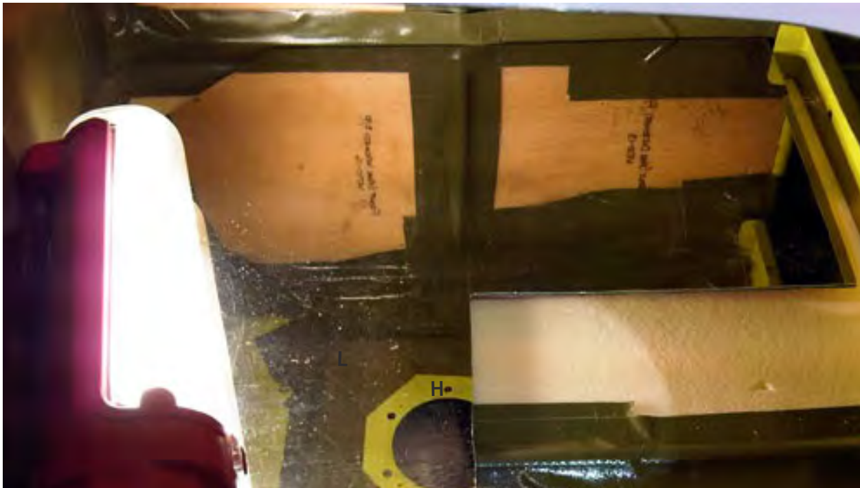
The bladder tank receives padding. Right wing is pictured here.
