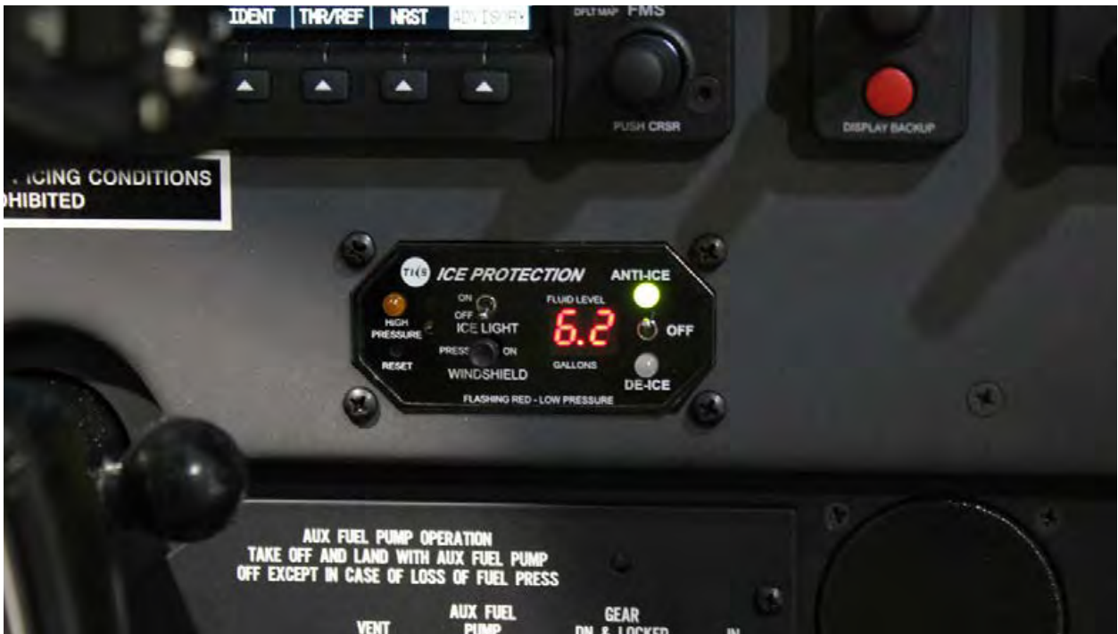
The TKS Ice Protection System Control Panel is adjusted and installed.
