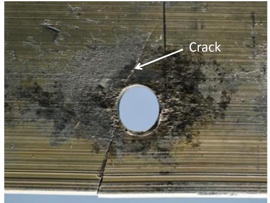
View of Spar Cap Lower Surface
